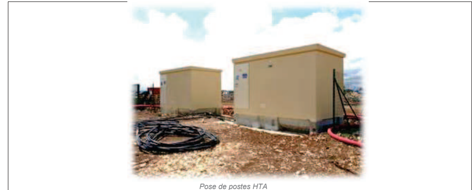
Pose de postes HTA
